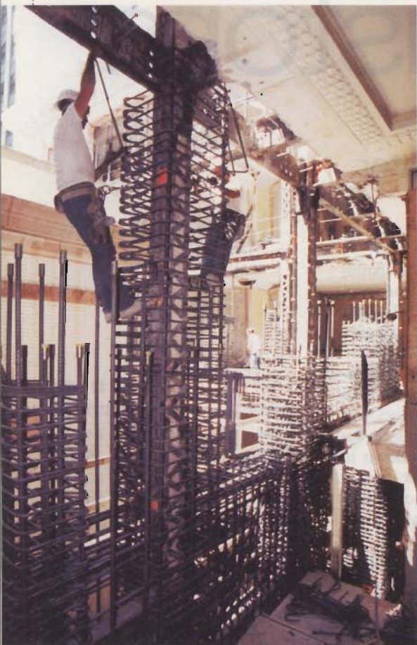
To provide lateral support, shear walls were installed around the building's perimeter. Courtyard walls (above) were completely demolished and replaced with cast-in-place concrete walls. The remaining perimeter walls (right) were demolished to their granite cladding from inside the building and replaced with shotcrete shear walls.
