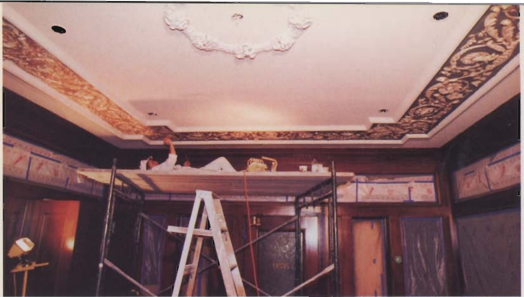
The historic finishes in the director's office include floor-to-ceiling wood and leather paneling and gilded ceiling plaster that were restored to their original specifications.
