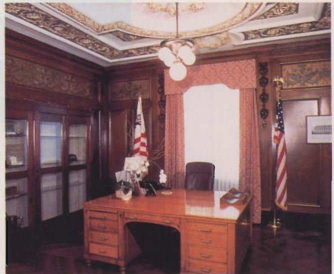
The historic finishes in the director's office include floor-to-ceiling wood and leather paneling and gilded ceiling plaster that were restored to their original specifications.
