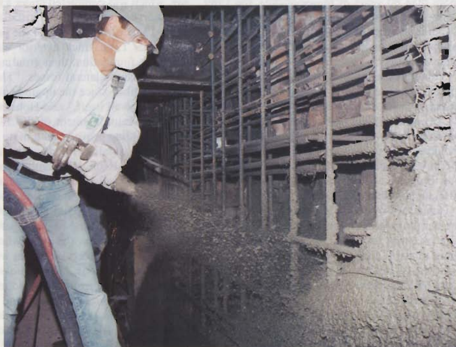
To provide lateral support, shear walls were installed around the building's perimeter. Courtyard walls (above) were completely demolished and replaced with cast-in-place concrete walls. The remaining perimeter walls (right) were demolished to their granite cladding from inside the building and replaced with shotcrete shear walls.
